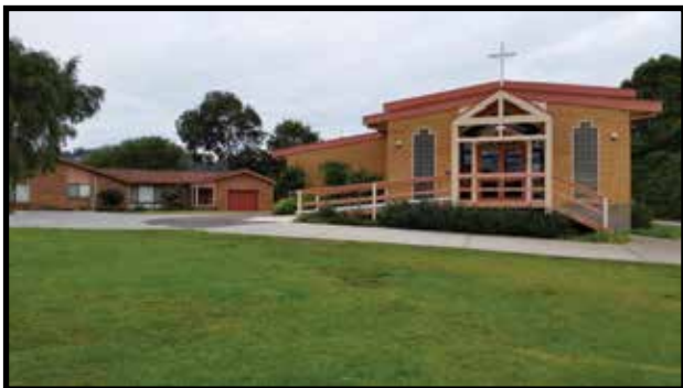
St. Clements Anglican Parish and Rectory
